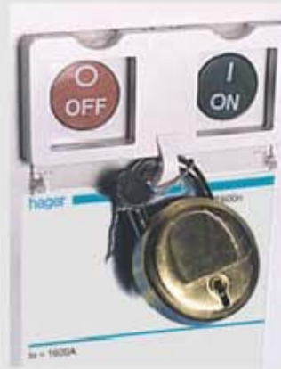
ON/OFF buttons can be sealed/padlocked.
